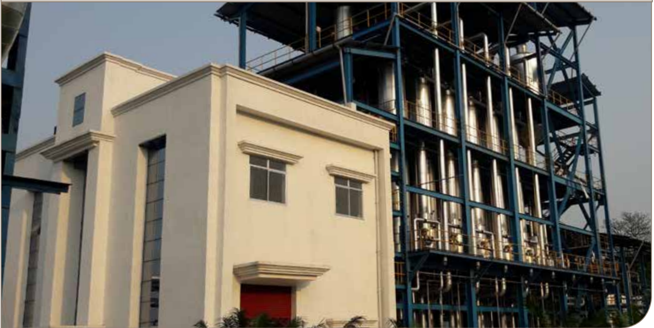
Degasification, evaporator and condensate polishing plant
